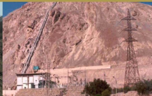
HIGH TENSION POWER LINES
